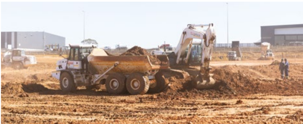
Precinct 2 bulk infrastructure development
